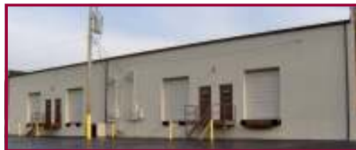
Loading Dock at Rear of Building
