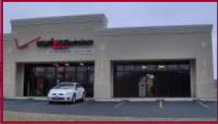
Northeast Building Elevation
