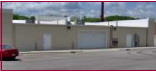
Well lighted Rear Access from Workman Road
