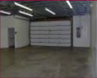
Potential Warehouse/Shop Entry
