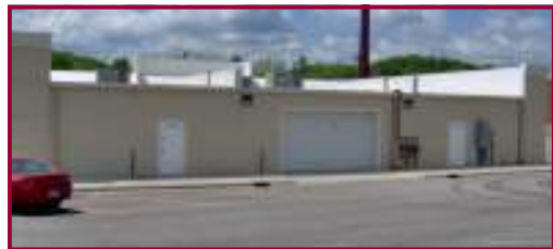
Well lighted Rear Access from Workman Road
