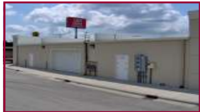
Rear of Building with Drive In Garage
