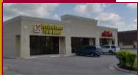
Northeast Building Elevation
