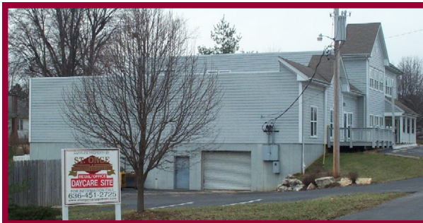
Drive in Door to Lower Level
