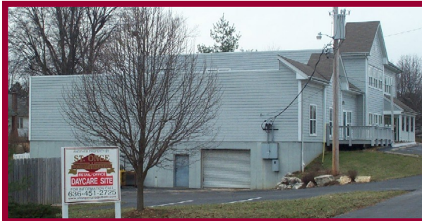
Drive in Door to Lower Level
